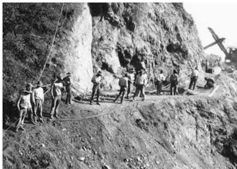
Beginning to widen the cut
