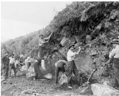
Starting to cut into the rock at Devil’s Elbow
