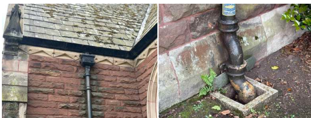
North transept – west side
