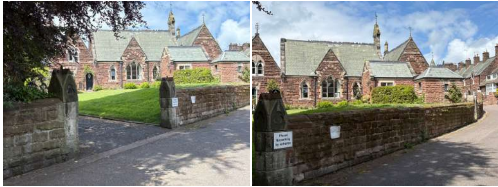
Northern boundary – the final photo shows a further section rebuilt in the quinquennium
