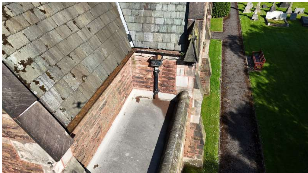
Gutter and short downpipe serving the organ and north transepts.
