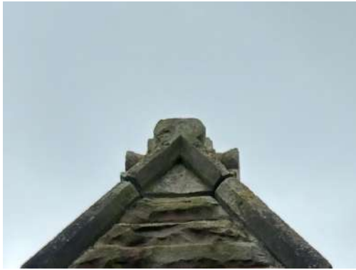
North transept - issues at apex stone and loose vent
