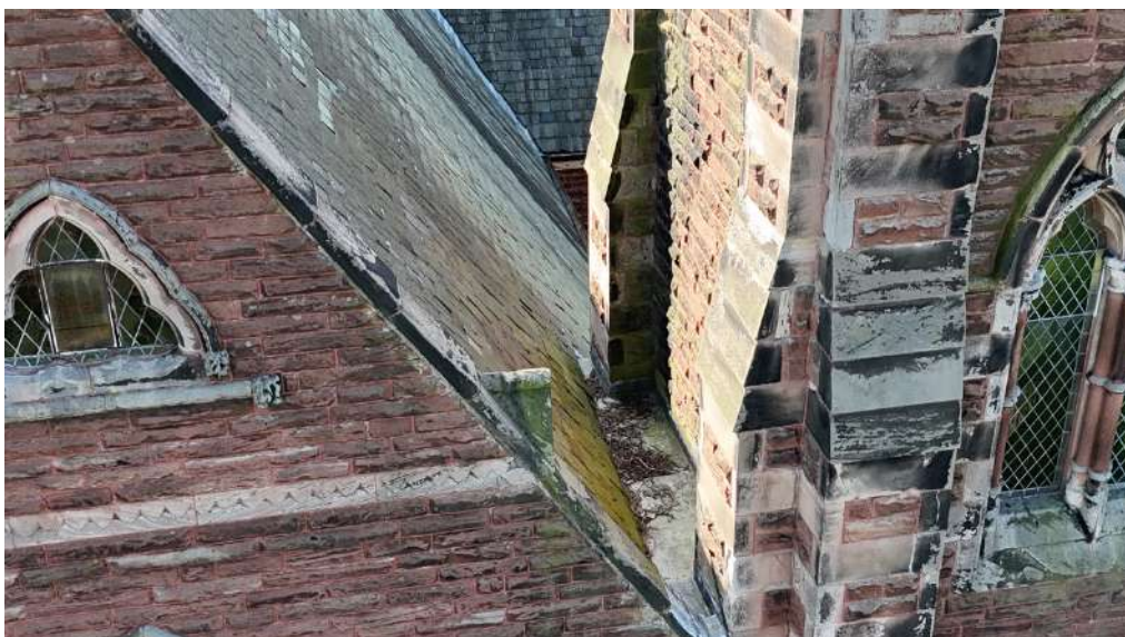
Lead gutter between the tower and south nave roof
