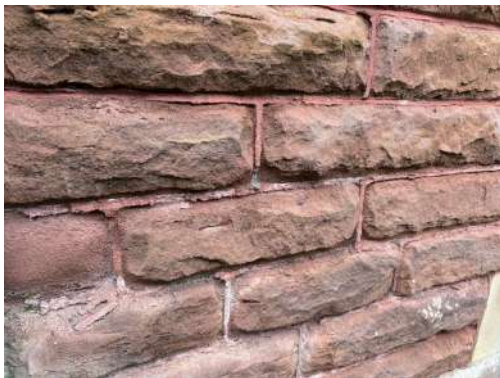
Choir vestry failing pointing and east side
