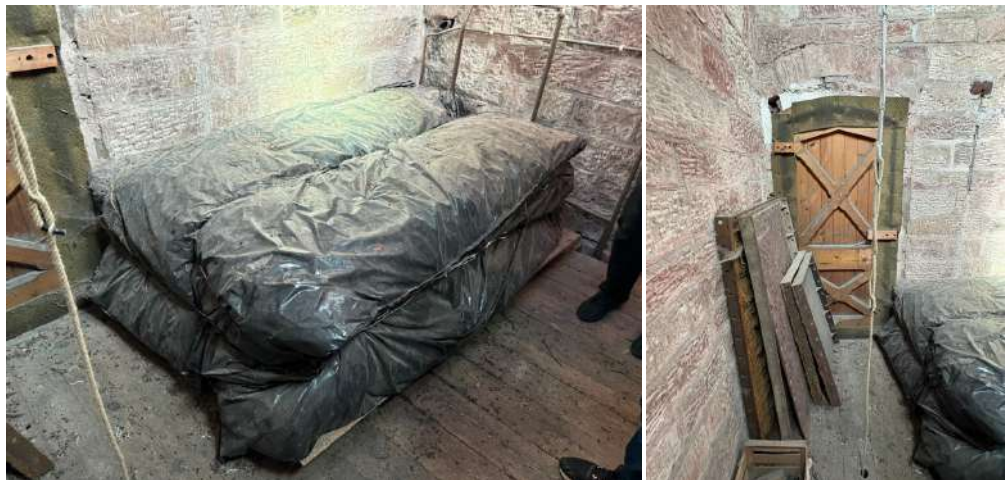
Sounding chamber – redundant tank and door to old gallery level
