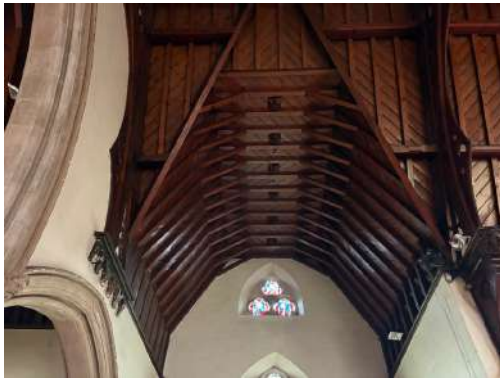
Transept ceiling and staining to the south side of the nave
