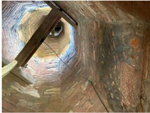
Interior of spire
