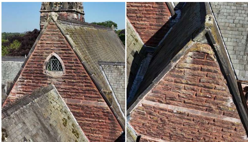
East nave and organ chamber transept gables viewed from a drone
