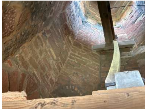
Interior of spire
