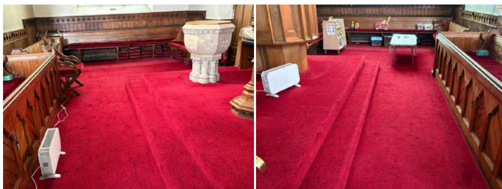
Flooring – front of nave / dais steps
