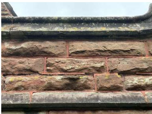
Choir vestry failing pointing on east side and deterioration around outlet
