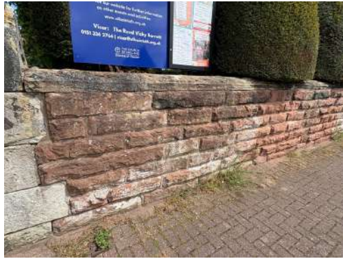
Areas of cracked and eroded wall
