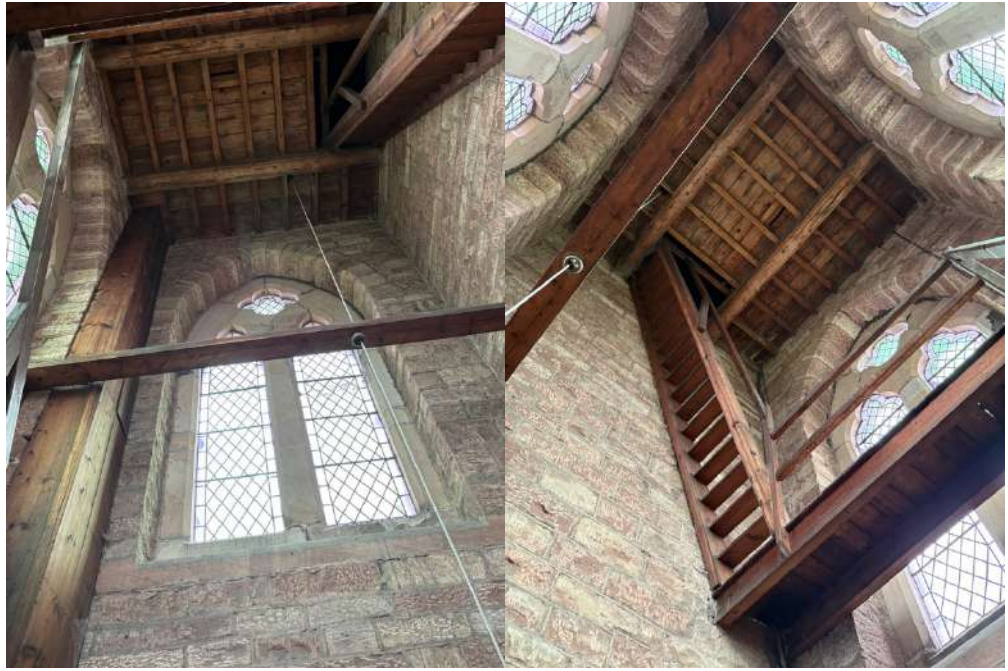
Ceiling of sounding chamber
