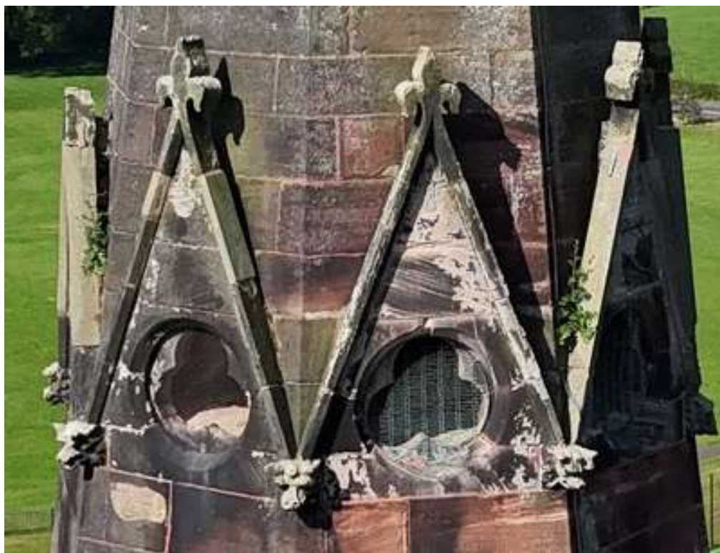
Plant growth on the north and north-east sides
