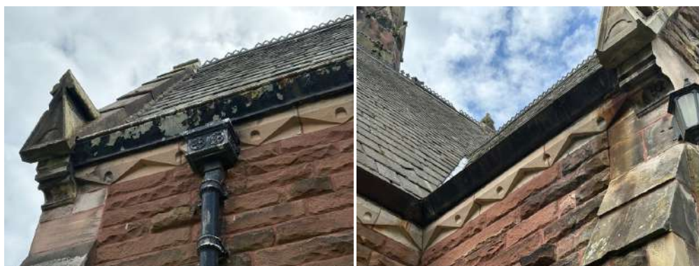
North porch rainwater goods
