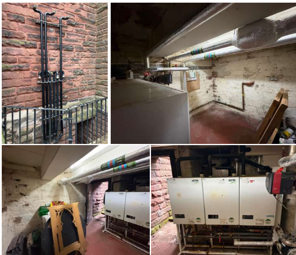
Existing boiler room and flues above the existing steps
