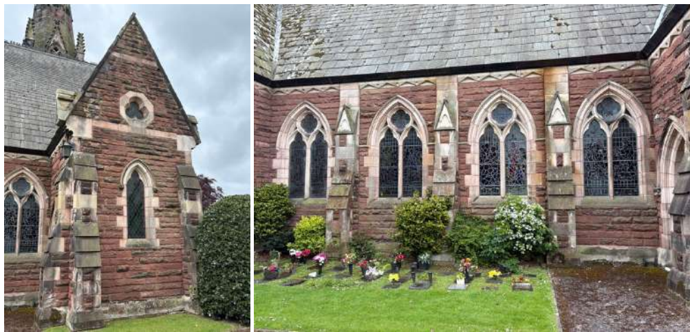
North porch and north nave elevations
