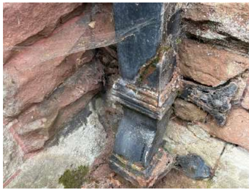
Choir vestry east- cracked downpipe and outlet into hopper
