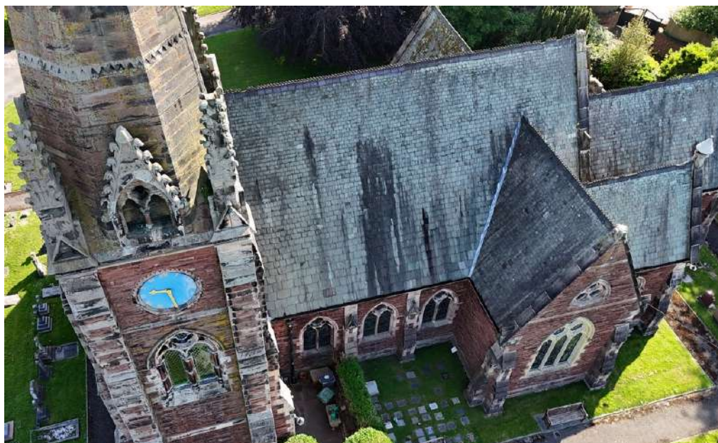
South nave roof
