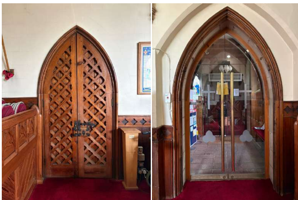
North and south porch inner doors
