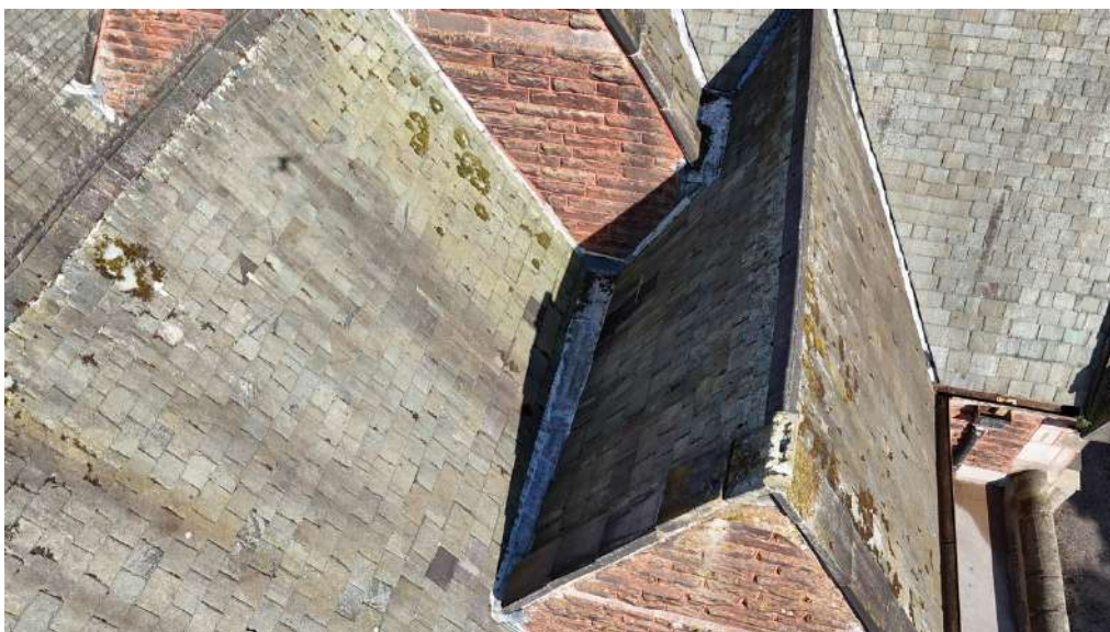
Vallet gutter between the organ transept and chancel
