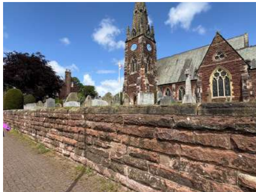
Area of minor lean and open joints (left) and more significant erosion
