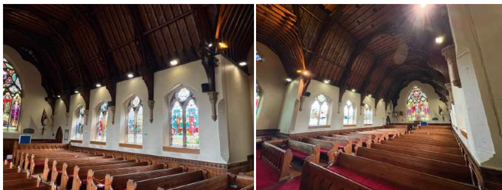
North side of nave and general view looking towards the west end
